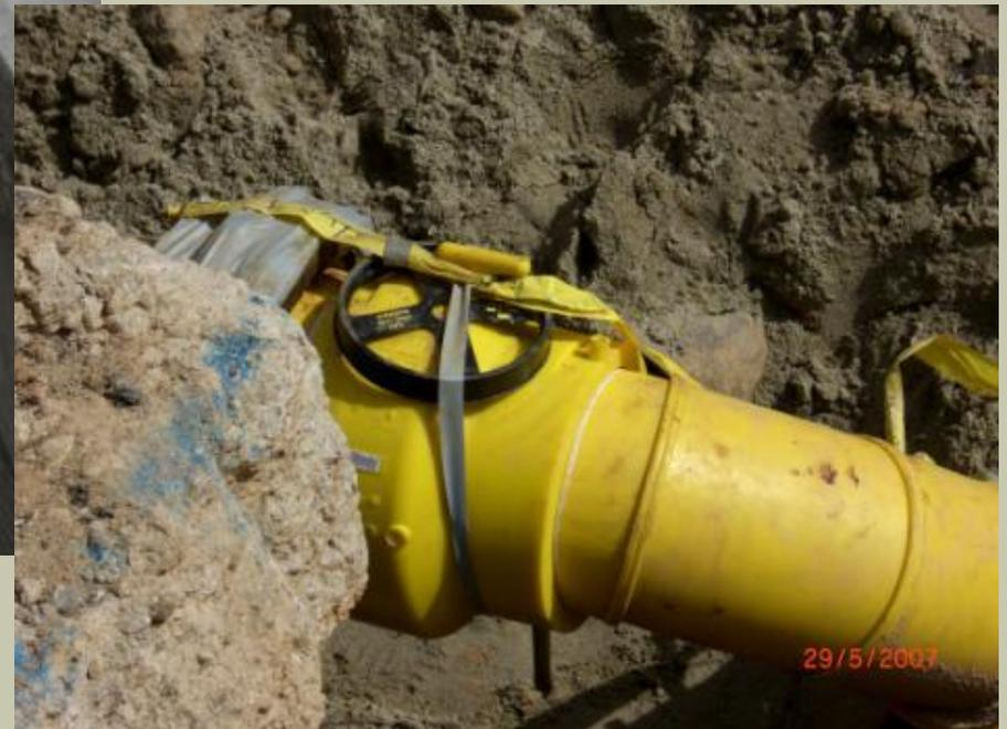
For Gas pipe without tracer wire
